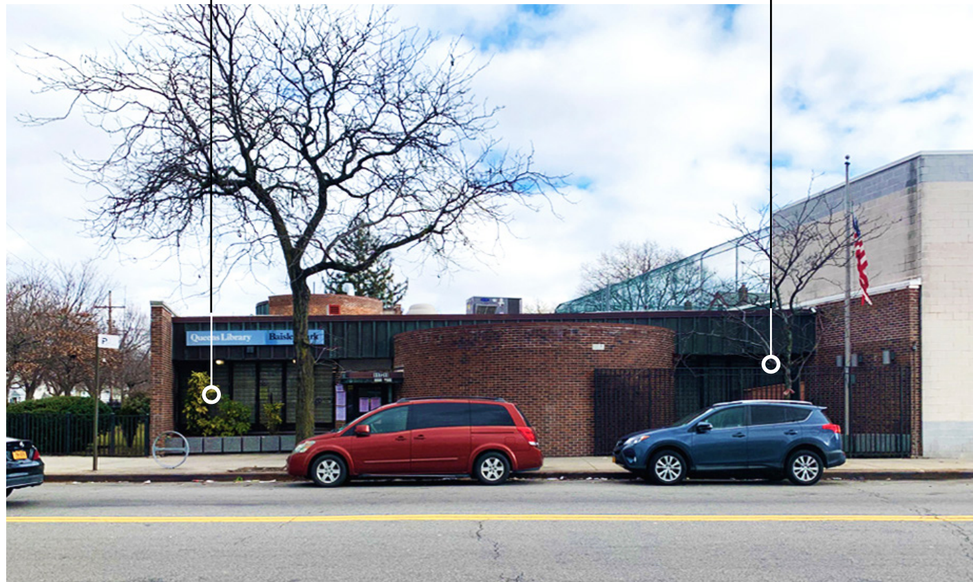
Existing Sutphin Boulevard Facade
